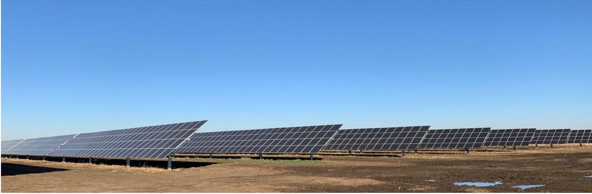
Figure 1 – Solar Arrays mounted on tracker systems
