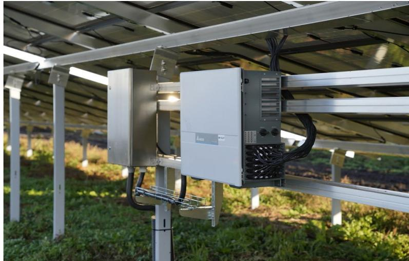
Figure 4 - Example of a string inverter, attached to the tracking array structure.
